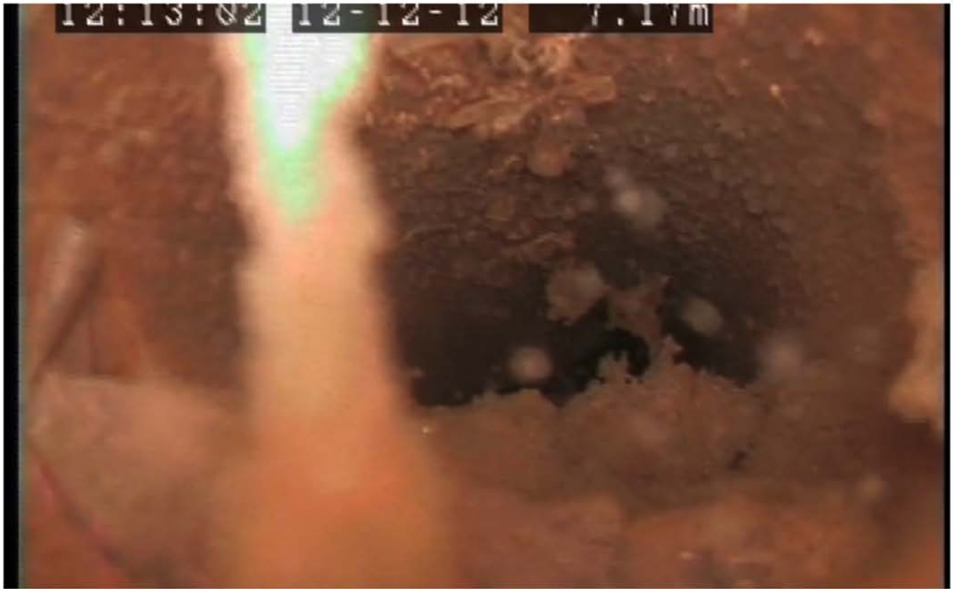
Example of the Typical Interior Conditions of the Pipes Before Cleaning
