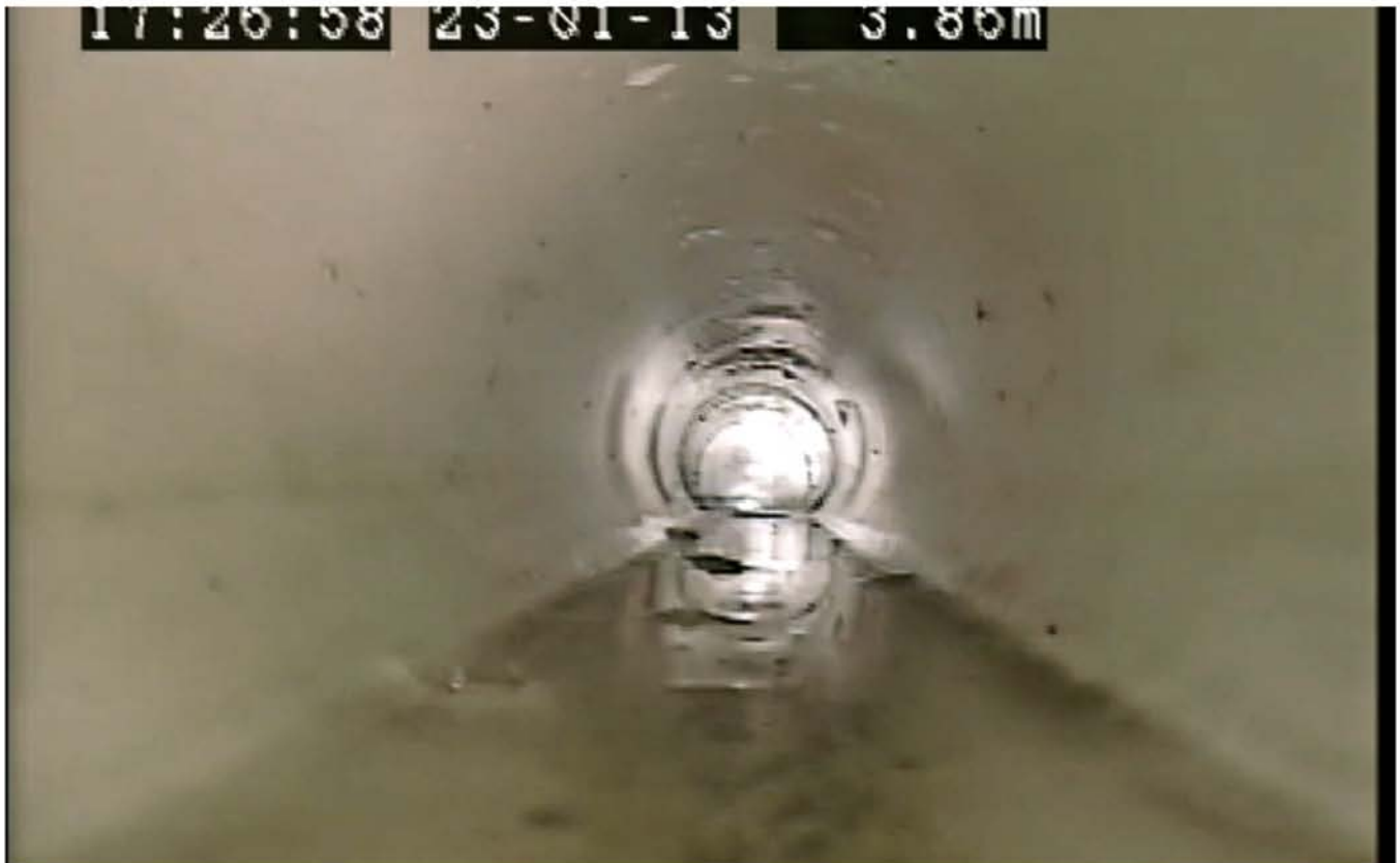
Example of the Typical Interior Conditions of the Pipes After Cleaning
