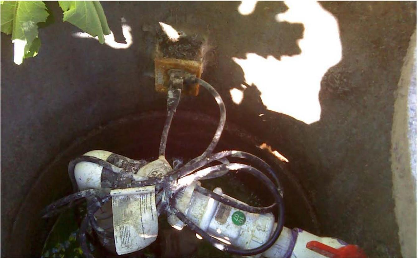
Interior of the Pump Chamber Showing the Electrical Connection
